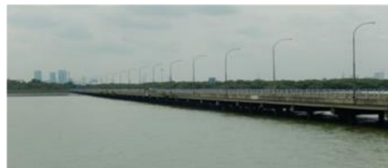
Figure 1. RC bridge investigated.
